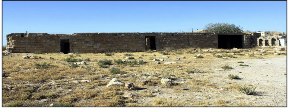
Nabulsi Building: Proposed site for the Hisban Education and Visitor Center.
